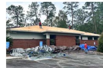
Construction on CCHD Roof
